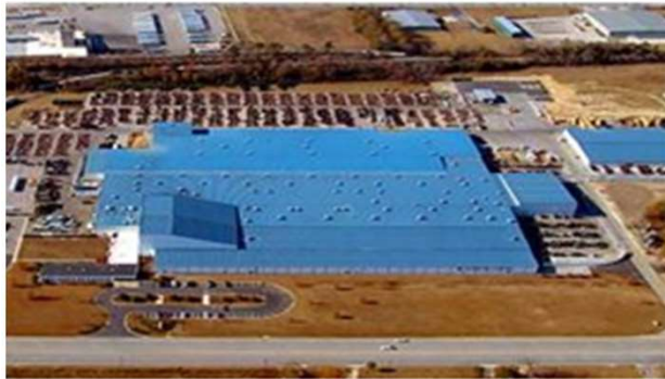
ORANGEBURG, SC (CABLE PLANT)
