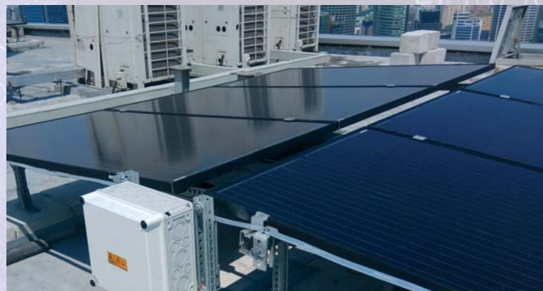
Numerous PV generator junction boxes are installed on the roof of the Marina Bay Sands Hotel.
