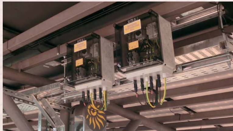
Numerous Hensel PV generator junction boxes ensure a reliable distribution of generated PV electricity.
