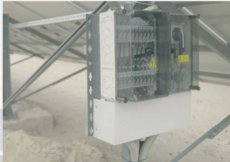
PV distribution boards close to a water source in the desert for a network-independent water pump system
