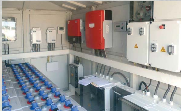
Electrification of a village in Liberia with PV generator junction boxes, PV power inverter collectors and battery distributors for protecting battery banks
