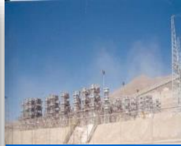
Minera Escondida Chile, 4400 meters, the world's largest copper mine
