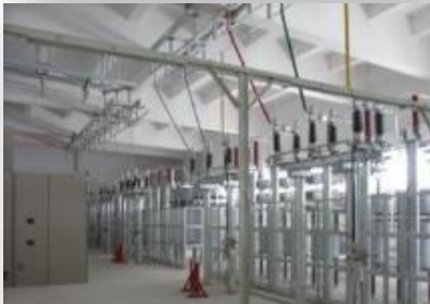
Lanzhou Aluminum Plant Filter system solution, 155MVAR
