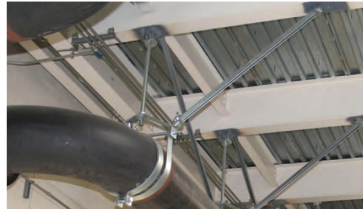
Seismic Bracing
